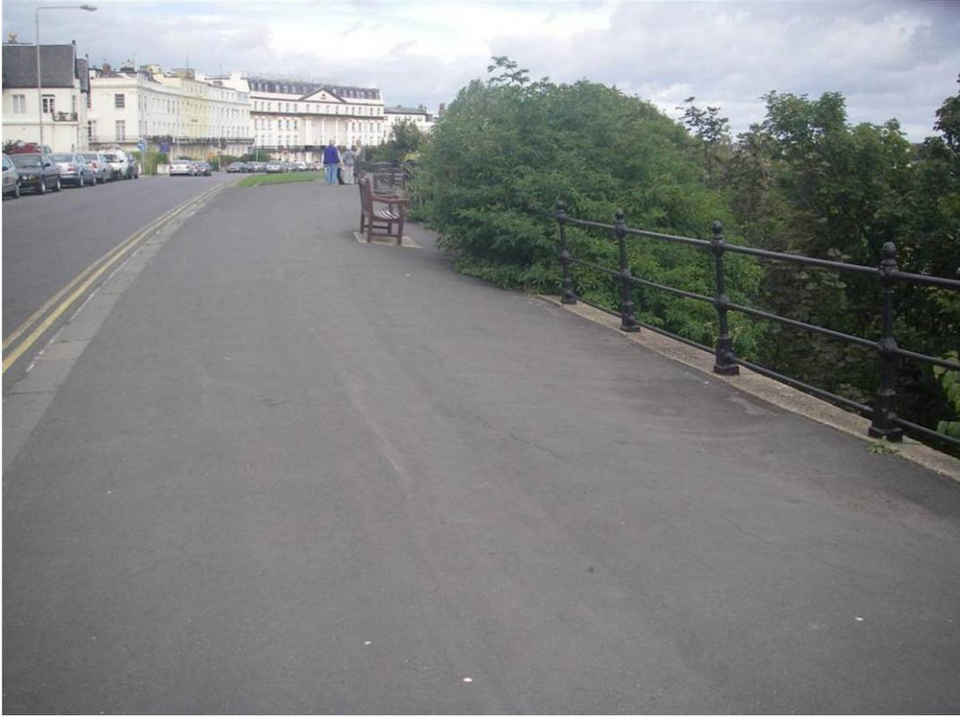
Plate 75 Scarborough South Cliff. Promenade showing signs of subsidence.
