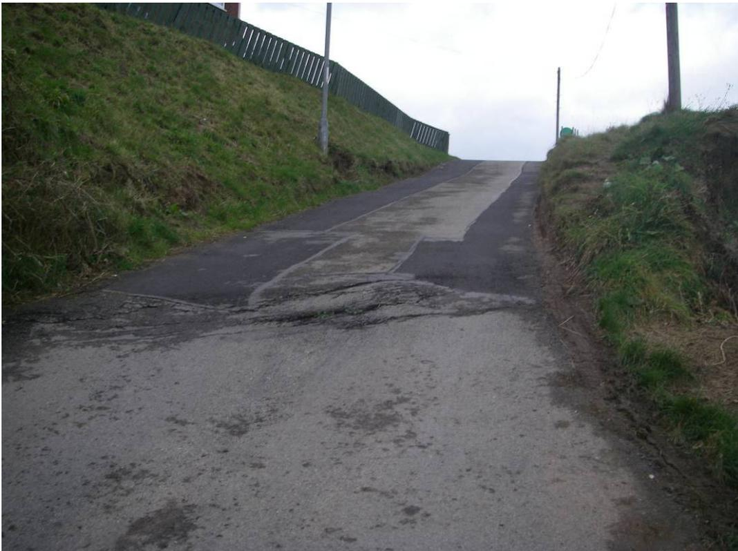
Plate 29 Site view of tension cracks and bulge in access road into Flat Cliffs.
